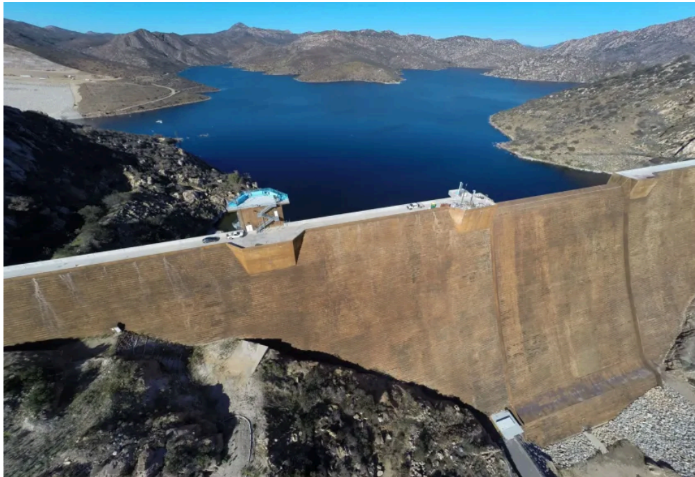
Dec. 29, 2014, San Diego, CA |Aerial view of the San Vicente reservoir which is set to re-open in 2015, letting anglers and water sports enthusiasts return to the lake which was closed seven years ago for raising the height of the dam more than 100 feet. (John Gibbins / The San Diego Union-Tribune)
